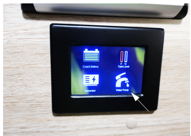
Water pump controls location on Systems Monitor Panel
