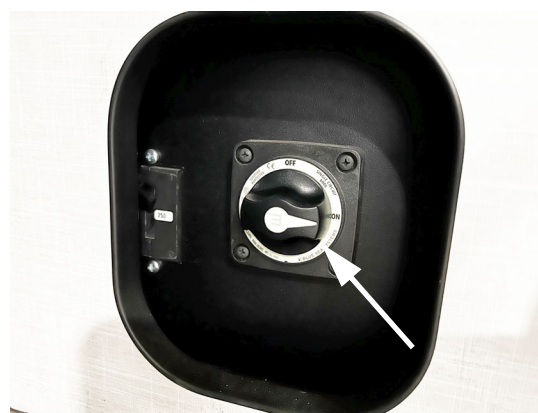
Inverter/charger disconnect switch. (Located on the side of the dinette seat) -Typical View
