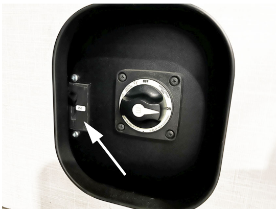
250 Amp circuit breaker (Located on the side of the dinette seat) -Typical View
