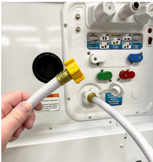
Antifreeze Siphon Tube attached to the tank fill inlet -Typical View
