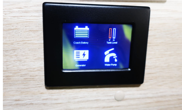
System Monitor Panel -Typical View
