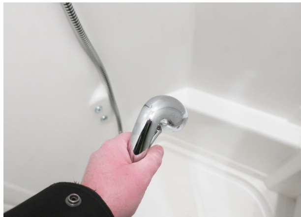
Point shower head at the drain and squeeze until water stops flowing. -Typical View
